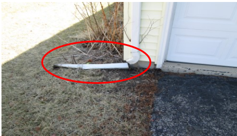
Broken downspout at ground level
