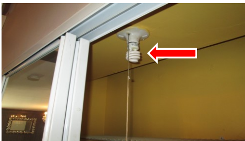
Light bulb cover is missing
