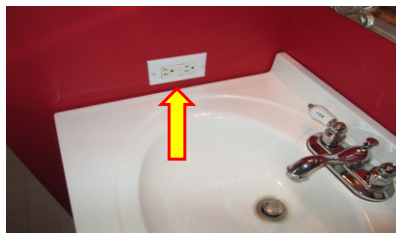
No GFCI / too close to water source
