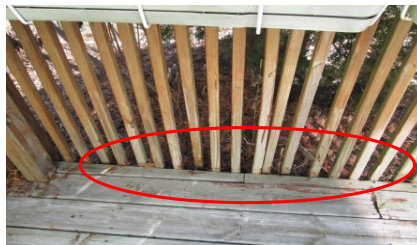
Loose and unsecured deck spindels
