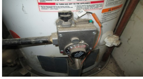
Dirty thermostat and gas valve
