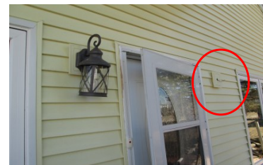
Light fixture missing
