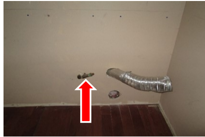
Gas supply pipe with shut off for dryer
