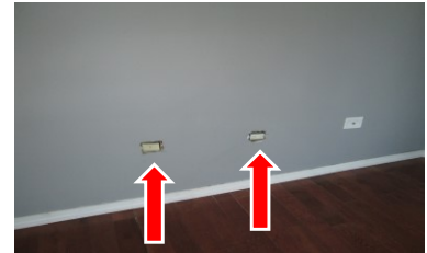
Cover plates are missing
