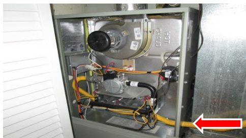
Flex pipe gas supply at furnace
