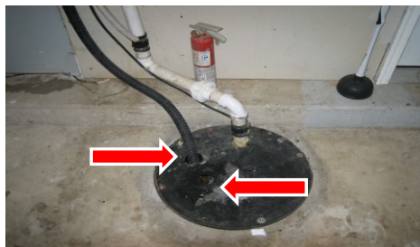
Sump pump with cover openings
