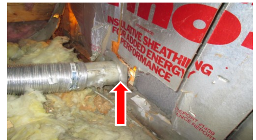
Dryer exhaust venting outside
