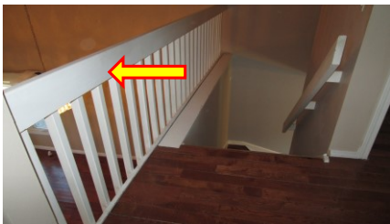
Guardrail not safe to lean on
