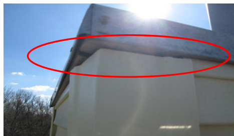
Unfinished Chimney top flashing
