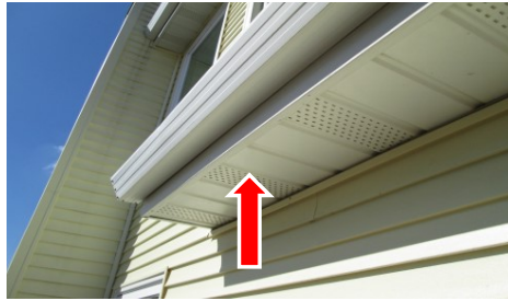
Soffit vents
