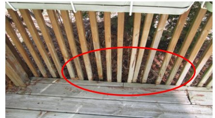
Loose guardrail mambers / unsecured
