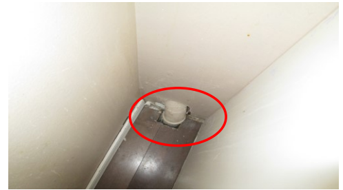
Every floor penetration must be sealed
