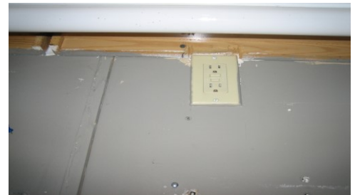
GFCI not working/ bad ground
