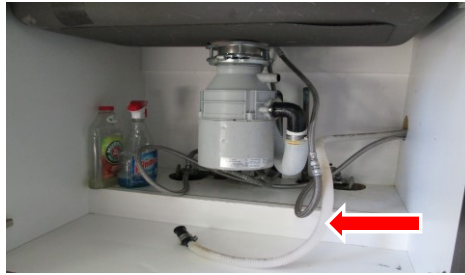
Kitchen plumbing/loose connector
