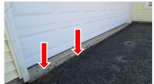
Low area where water is pooling
