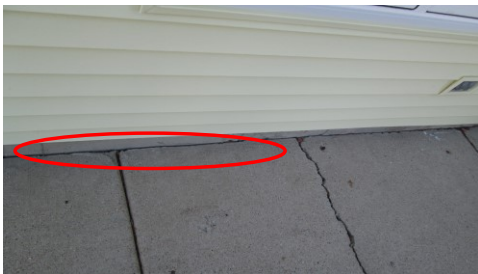
Gap between walkway and fundation
