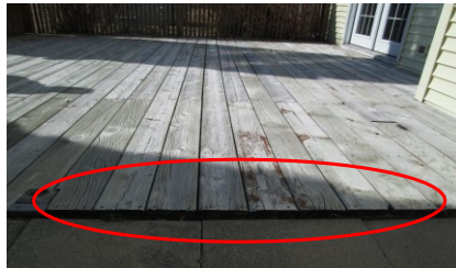
Trip hazard from wood deck to pavers
