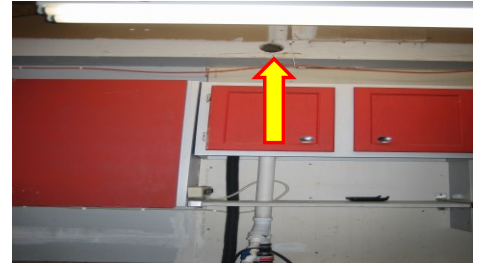
Holes in garage-house common wall
