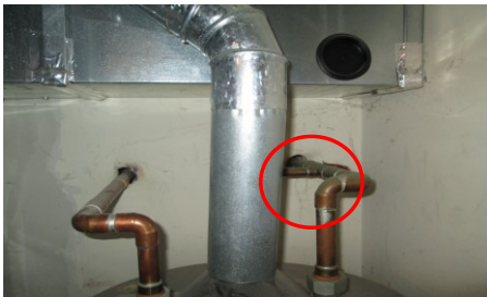
Cold water shut off
