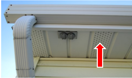
Soffit vents
