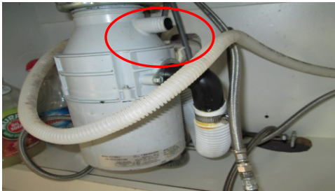
No connection / open water outlet
