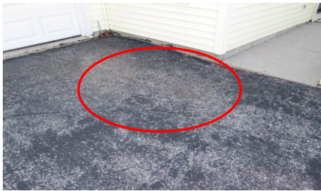
Low area where water is pooling
