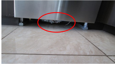
Dishwasher electric wires are loose
