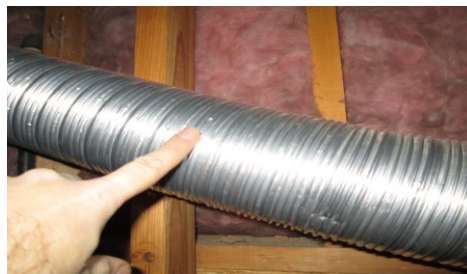
Dryer exhaust /negative pitch
