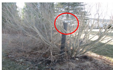
No GFCI and weatherproof cover
