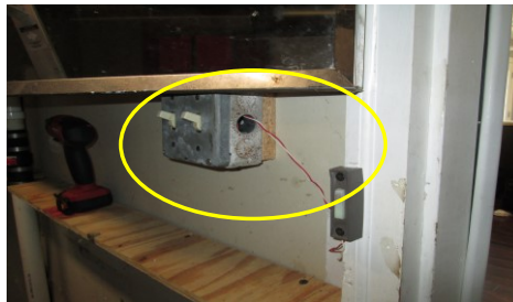
Illegal connection and open knockout
