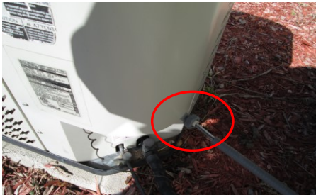
Exposed electric wires
