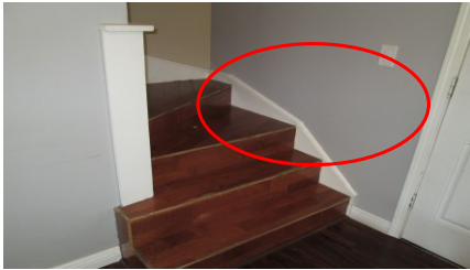
Handrail missing
