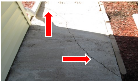
Crack on walkway
