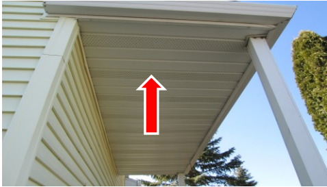
Soffit vents
