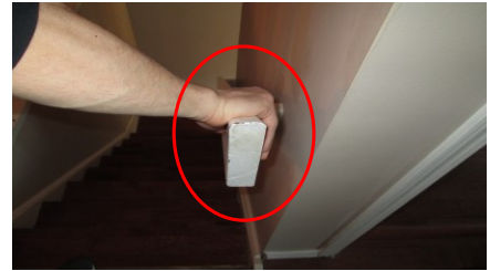
Handrail hard to grab and hold
