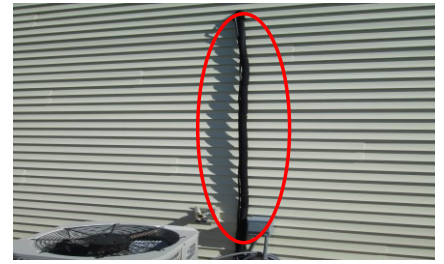
Refrigerant lines are weathered
