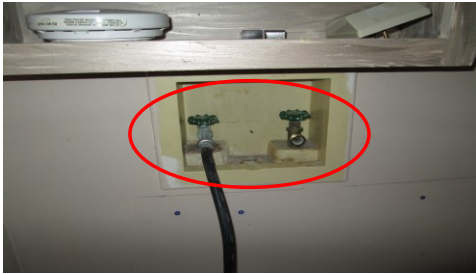
Washing machine water supply
