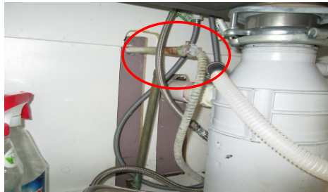
Wrong electric connection
