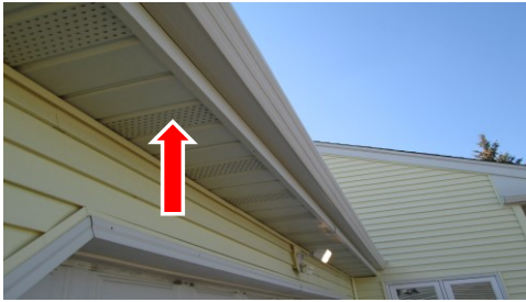
Soffit vents
