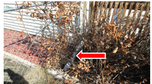
Broken downspout at ground level
