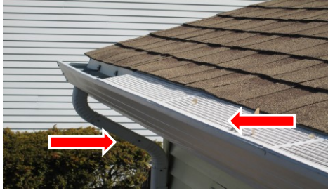
Gutter and downspout
